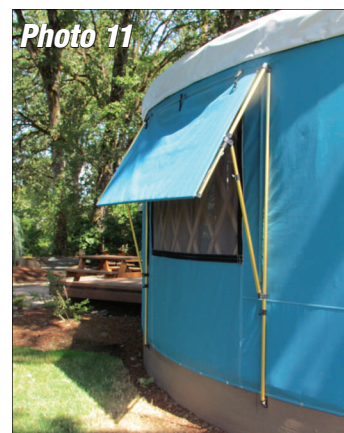
Extended Window Awning Frame
