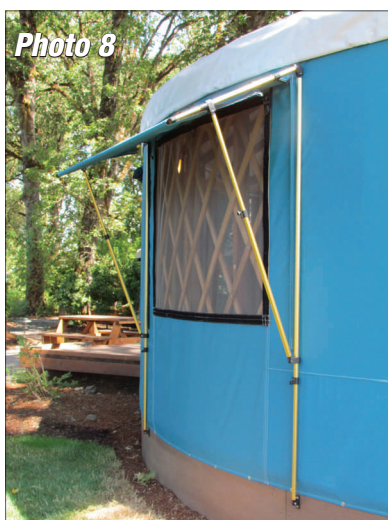
Completed Window Awning Frame
