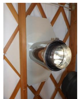
7. Install the woodstove on a fire-proof base **following the stove manufacturer's guidelines for specific clearances from combustible surfaces**. Single-wall stovepipe can be used up to the exit flashing, where a Metalbestos or equivalent (insulated) pipe is inserted through the flashing to safely vent the hot gases through the side cover.
