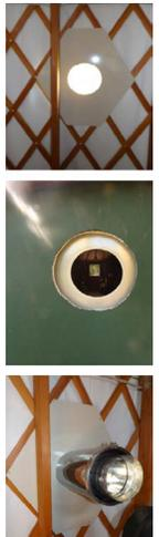
**The Pipe:** The stovepipe through the wall and any exterior piping should be insulated pipe that is rated at 2" clearance from the nearest combustible surface.
