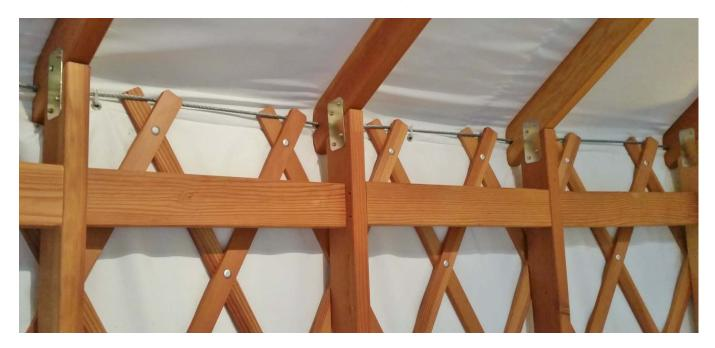
Perimeter blocking may be installed after the entire yurt has been installed or during the installation (immediately after the rafter supports are installed). This blocking is essentially 2x4 blocks fastened horizontally between the rafter supports and door(s). It creates a secondary 'compression ring' near the top of the wall, so it is important that it be continuous. Do not omit blocks next to the doors.
